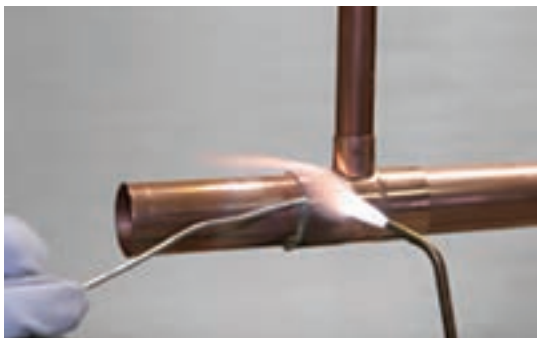
SOLDERED JOINTS
